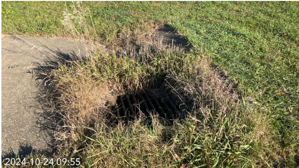
Photo Location 27. View of storm drain. Photograph taken facing north.
