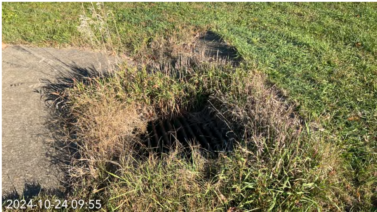
Photo Location 27. View of storm drain. Photograph taken facing north.
