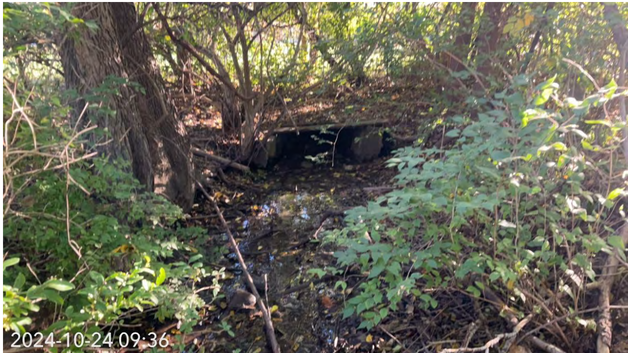
Photo Location 26. View of Stream 01 (Intermittent) flowing through culvert. Photograph taken facing downstream, east.
