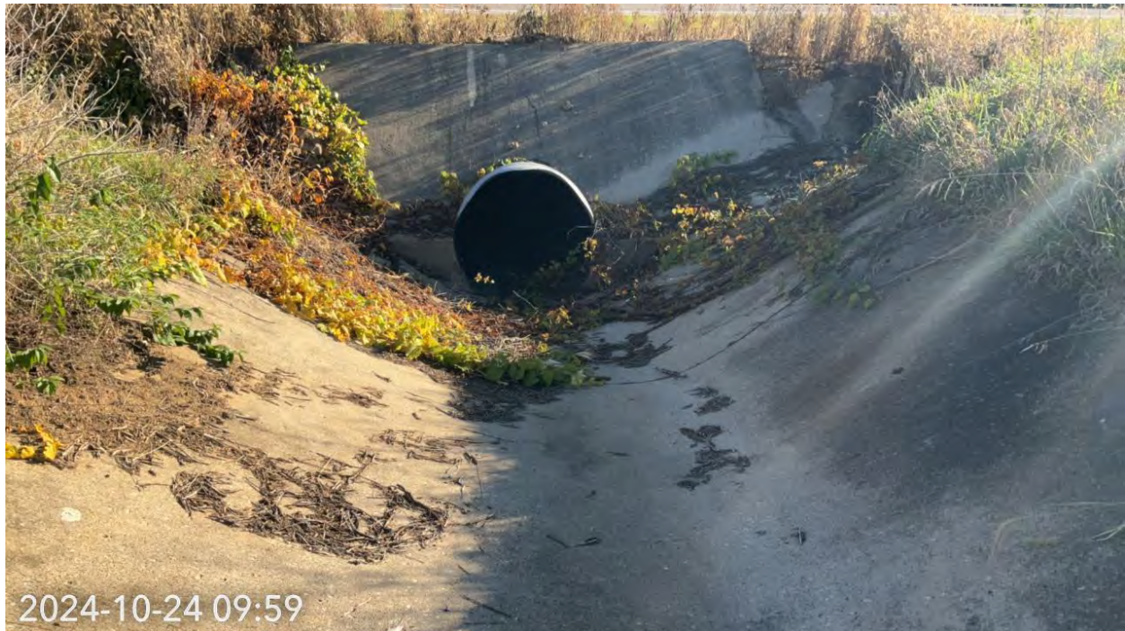
Photo Location 32. View of concrete channel and culvert. Photograph taken facing east.
